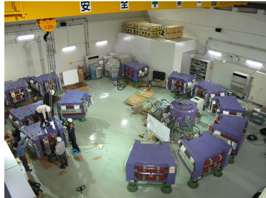
4. Alignment of the main ring (Jun - Dec 2009)
