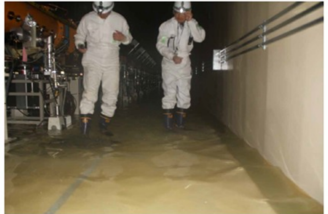
Linac Tunnel as of March 24
